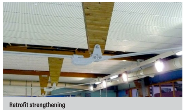
Wall Panel Tie-back
