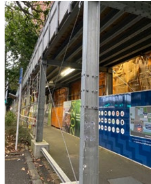
Temporary Work / Platform Bracing
