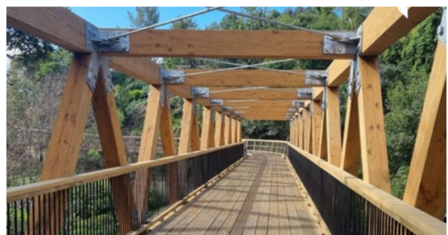
Timber Structure Bracing
